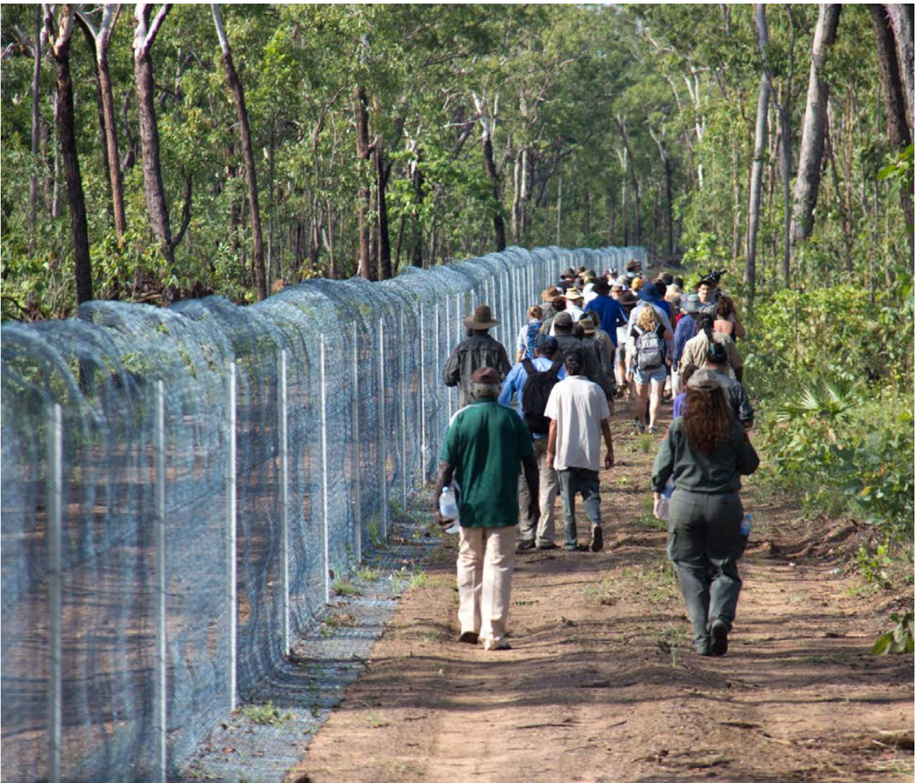
This cat enclosure fence was completed in Kakadu in late 2013.
