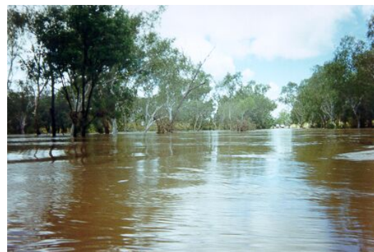
Waterhouse Creek Crossing in flood.
