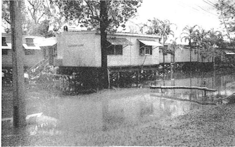
The Christian Leadership Centre at Five Mile, Daly River after the 1998 flood. Normally when floods threaten this is the place to which vehicles and people are evacuated. It is normally above the flood level.
