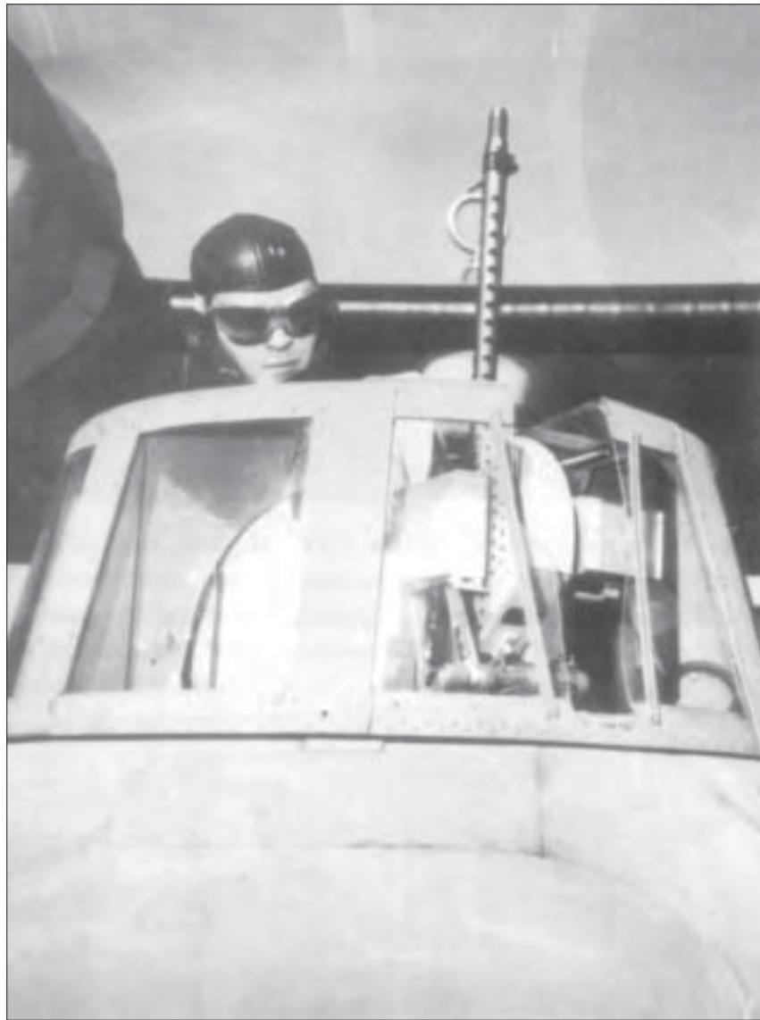
Photo 13. The standard type gun turret on pre-PBY-5A Catalina types with the single .30 in. calibre machine gun (Kinzey 2000:56).
