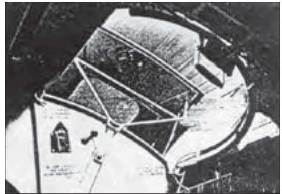
Figure 9. 'Five views of the two decks gun positions. On the left the portion of decking which protects the gunner from the airstream is shown being raised after having been slid forward. The third view shows the side plates in position. Below is a "shot" of the gunner's position from inside the hull and below that is a view showing everything ready for action, except that the gun is not fitted to the track-type mounting which, incidentally, operates very smoothly' (Flight 1939:b).
