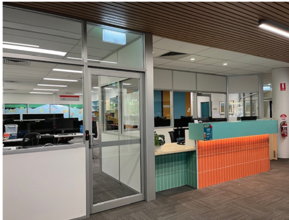
Figure 3. Reused aluminium partitions.
