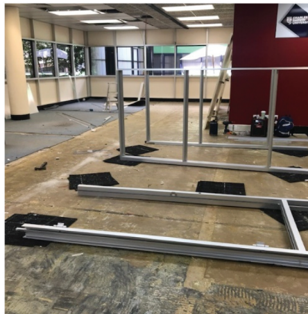
Figure 4. Careful dismantling of aluminium frames.
